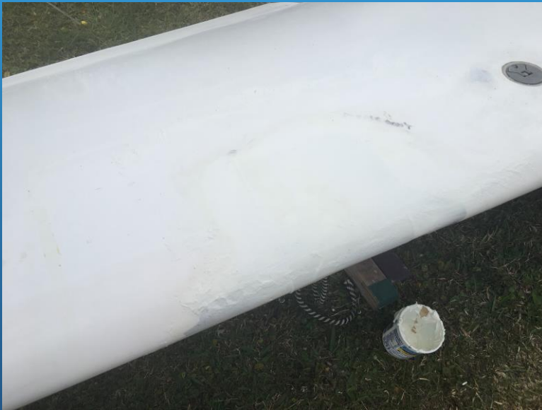
Dry micro to fair the repaired area.
