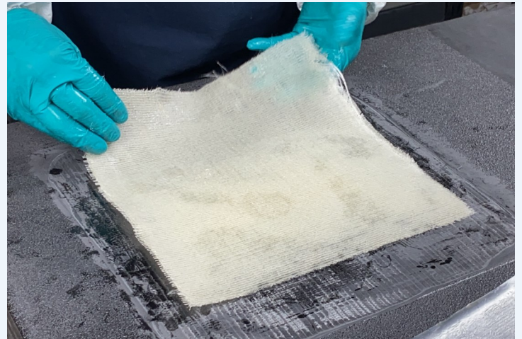
4 The glass fiber/vinyl ester repair patch is cut to size and positioned on the repair area.
