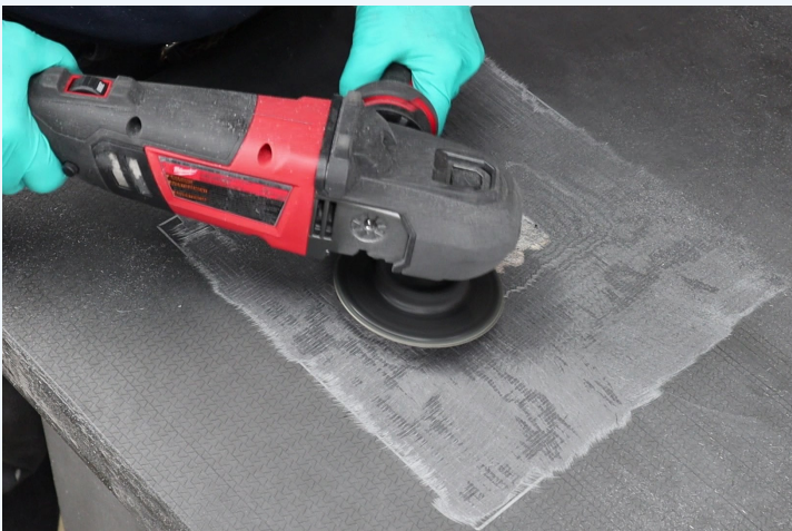
2 A battery-powered hand grinder is used to remove damaged material and scarf a 12:1 taper to receive the repair patch.
